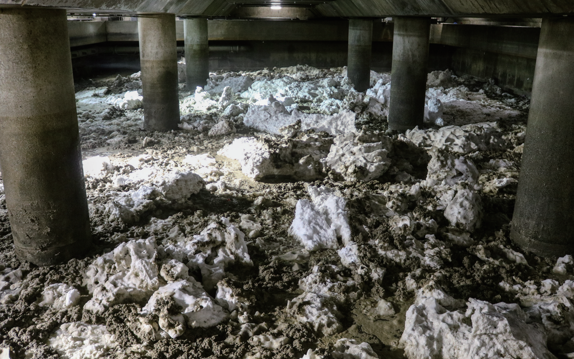
都心北融雪槽 Snow-melting tank
